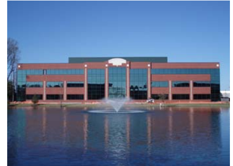
Liberty III, Chesapeake, VA LEED Silver certified
