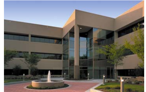
One Independence Point, Greenville, SC LEED-EB Certified
